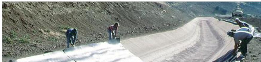
Figure 1: installation of the liner in 1993
