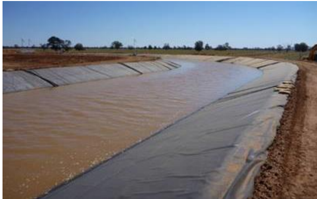
Figure 1. Irrigation canal in Australia – Earth canal renovation
