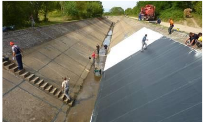
Figure 2. Canal for Hydroelectric production in Serbia – Concrete canal renovation
