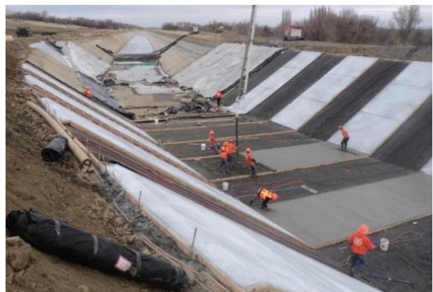
Figure 2: Installation of concrete on a geomembrane
