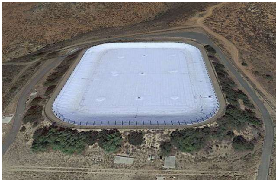
Figure 7. Aerial of Upper Reservoir CSPE Cover
