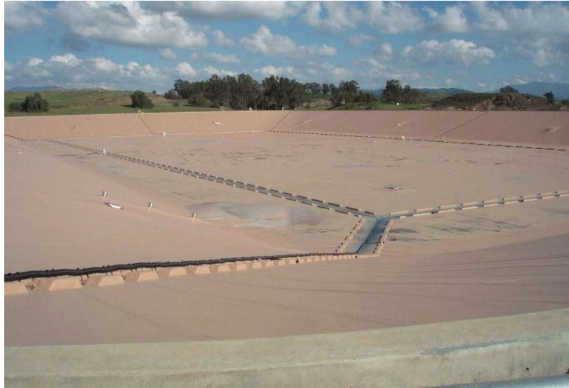
Figure 4. MWDS Skinner Reservoir, CSPE Cover installed 2010
