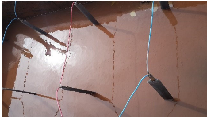
Figure 4. New drainage product installed in pool number 4
