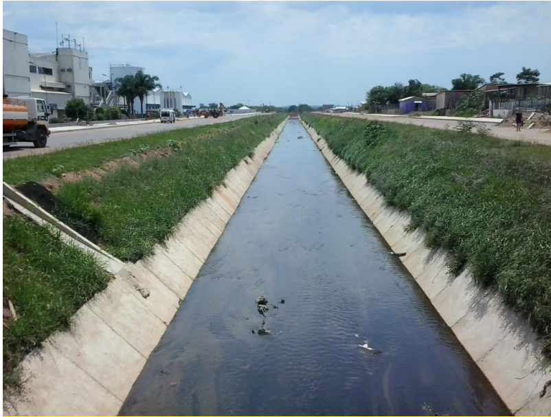
Figure 9. View of the work completed in August / 2014.
