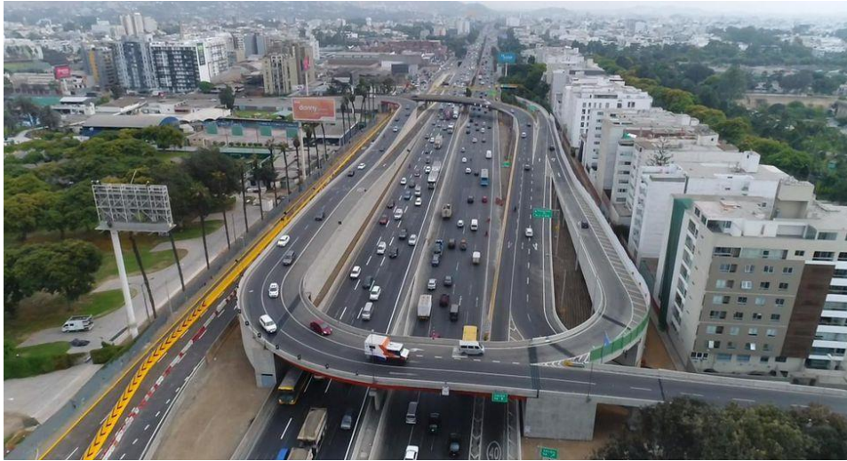
Picture N°7. Reinforced Soil Wall – RI (Road Interchange) “El Derby”
