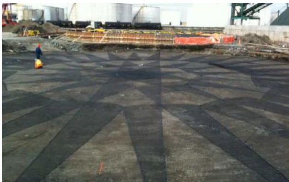
a) Geogrid reinforcement on excavation base
