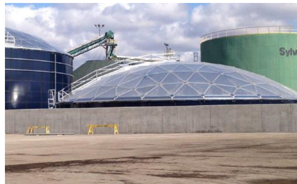
b) Tank built on geogrid-reinforced ground mass
