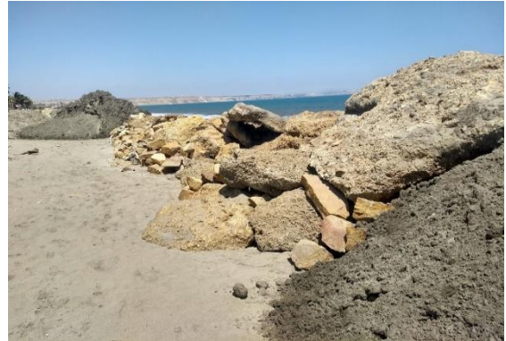
Figure 11 and 12. Provisional sand and rock barrier next to the Geobags.
