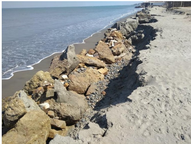
Figure 14. Sand and stone barrier wash produced by the tide.
