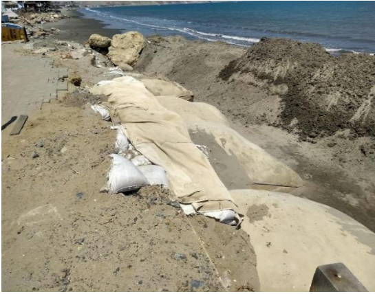
Figure 11 and 12. Provisional sand and rock barrier next to the Geobags.
