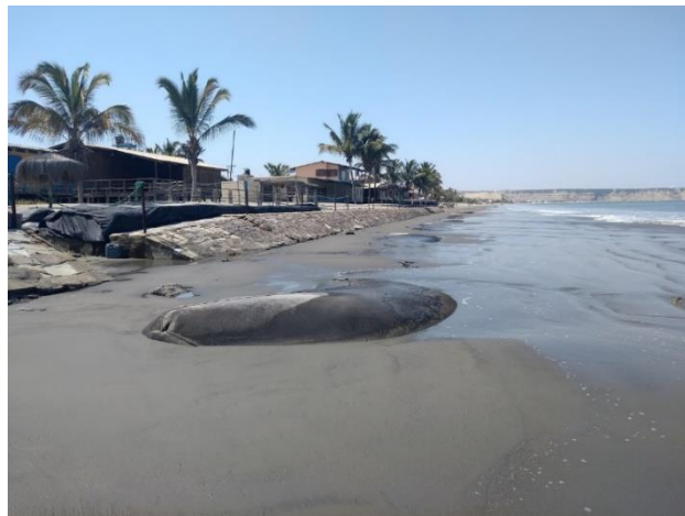
Figure 16. Geobags in areas near the resort.
