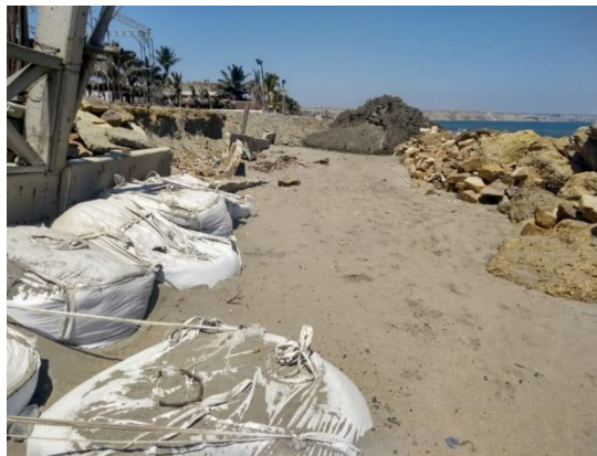
Figure 1. Geobags used in the coastal defense of the Costa Bonita resort.
