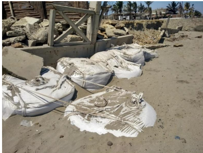
Figure 8. Geobags covered by sea sediments.
