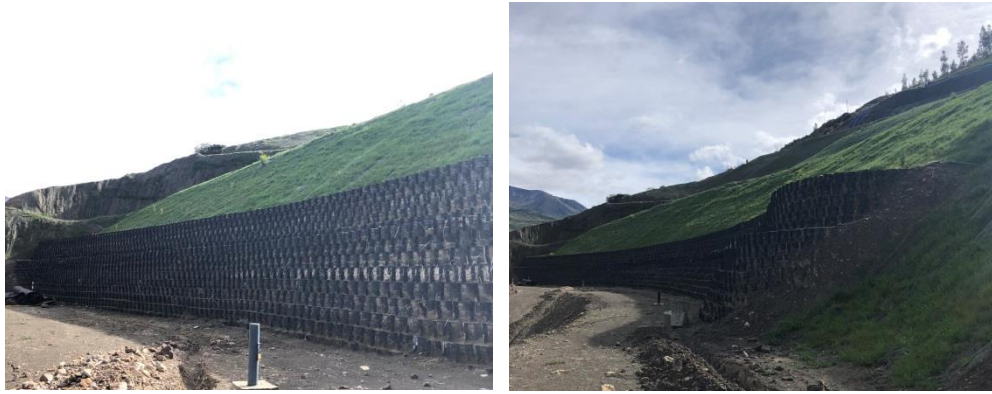
Figure 11. Front view in operation
