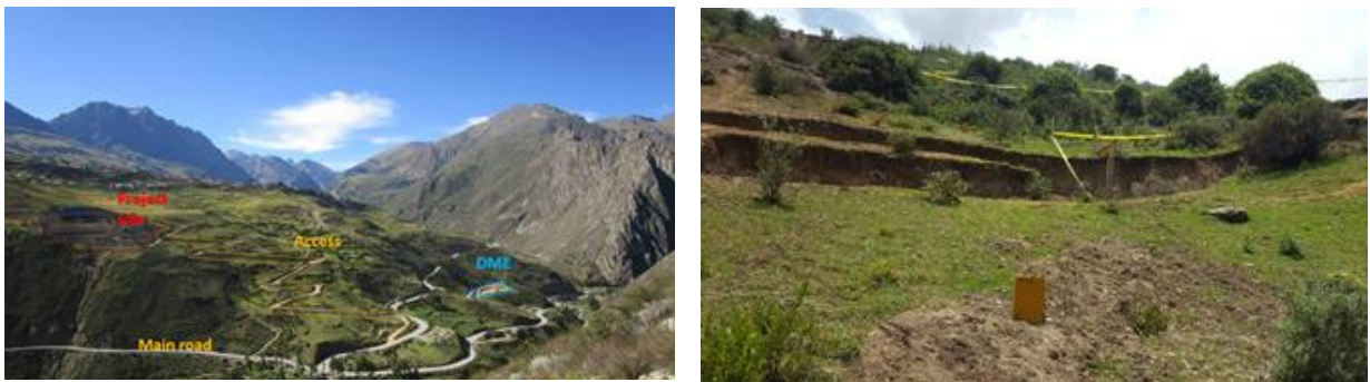
Figure 2. Overview of the project site (left) and the steep irregular slopes (right)
