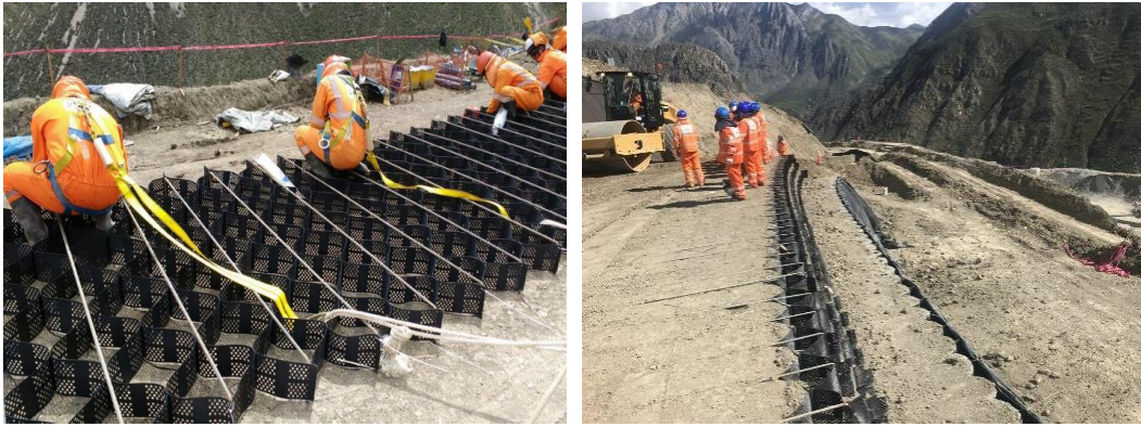
Figure 7. Expanded geocells with steel bars and filled with structural fill soil
