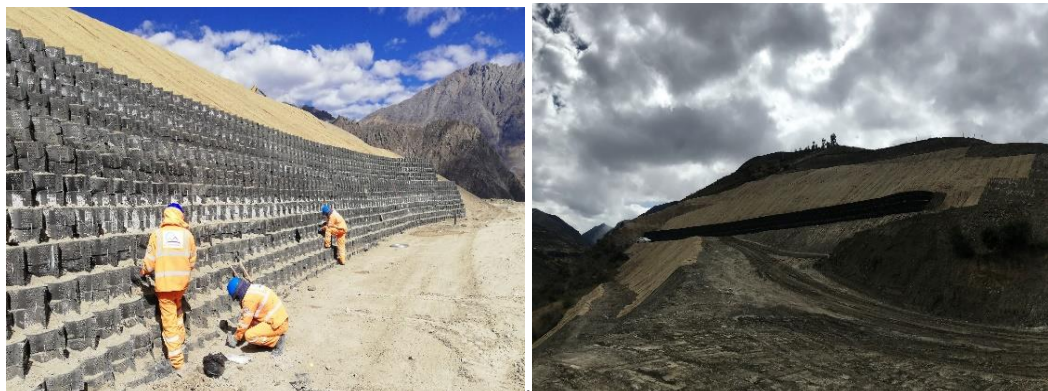
Figure 10. Front view of the end of the construction
