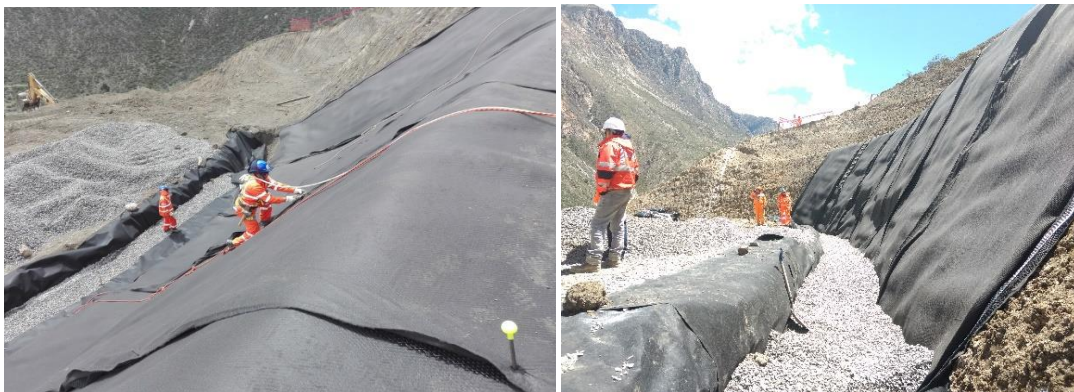
Figure 9. Laying drainage blankets
