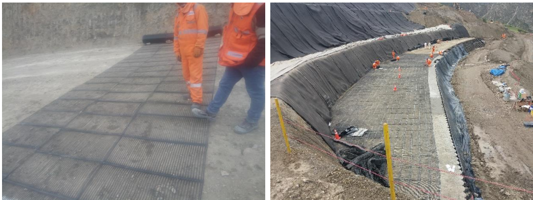
Figure 8. Laying of reinforcement geogrids
