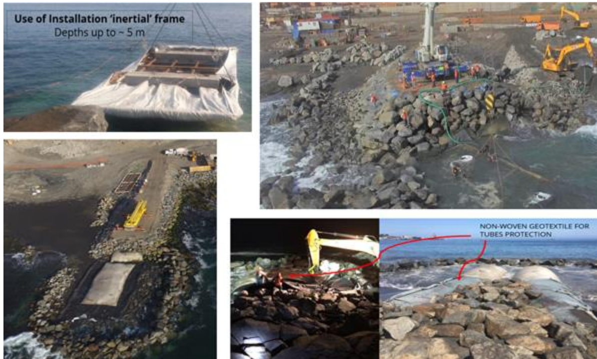
Figure 3. Construction detailed sequence.
