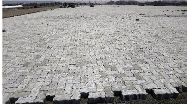
d) Laying of Paver blocks to finish the surface
