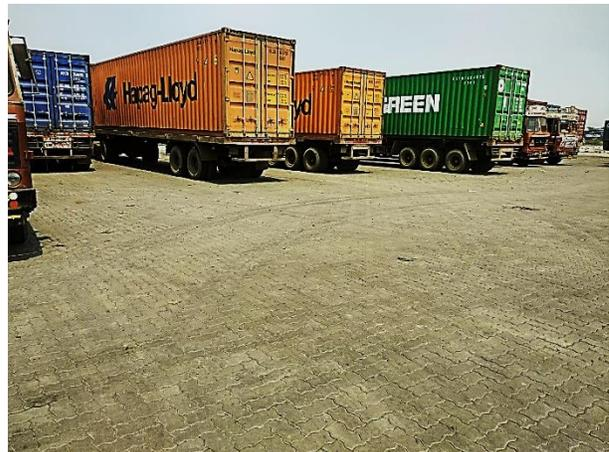
Figure 7 The paved surface including turning circles with heavy container carrier traffic, after 18 months of operation
