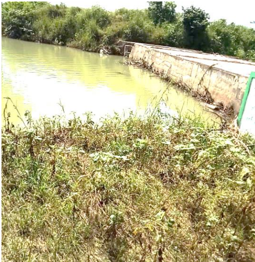
a) Upstream of check dam after the second monsoon - 2019 (1.5 years post construction)
