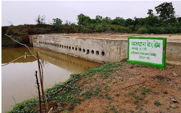
a) Upstream of check dam after the first monsoon - 2018 (6 months post construction)
