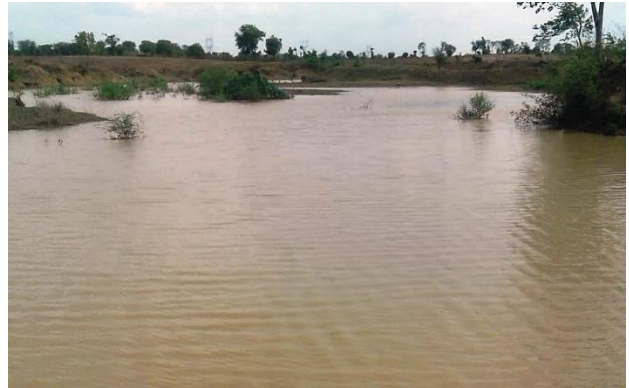
b) Reservoir behind the check dam after the first monsoon - 2018 (6 months post construction)
