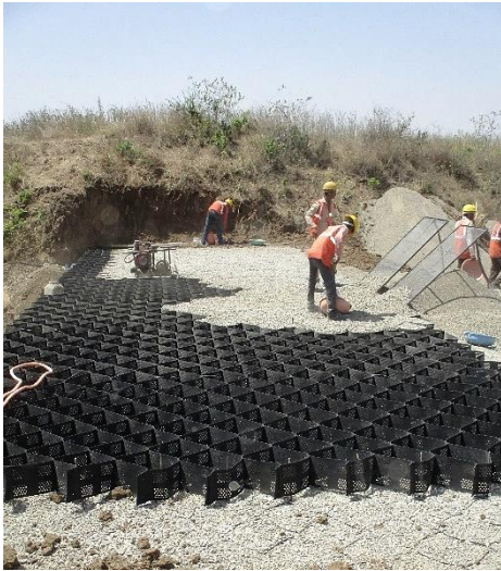
Figure 5. Infilling of geocells with non-plastic material
