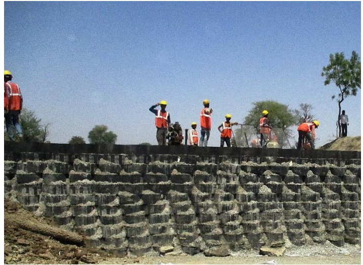
Figure 6. Construction of check dam up to spillway level
