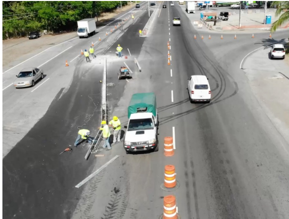
Figure No.4 Prior to resurfacing
