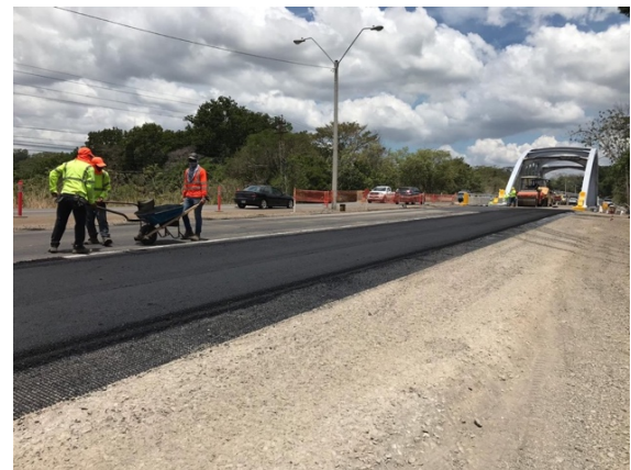
Figure No.7 After the fiberglass geogrid and new asphalt binder
