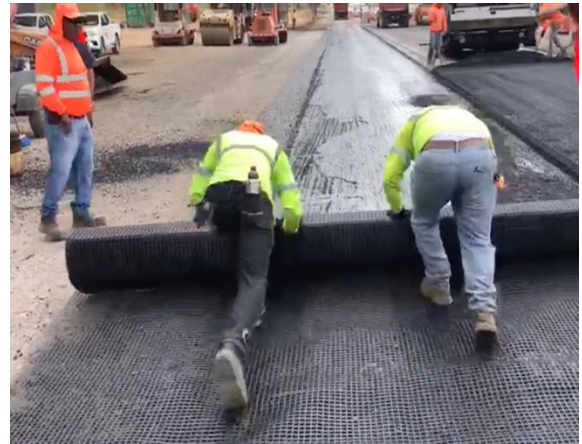
Figure No. 5 Manual placement of the fiberglass
