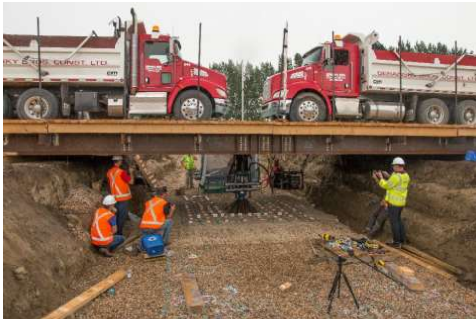
Figure 3: Constructed steel load platform with loaded gravel trucks above
