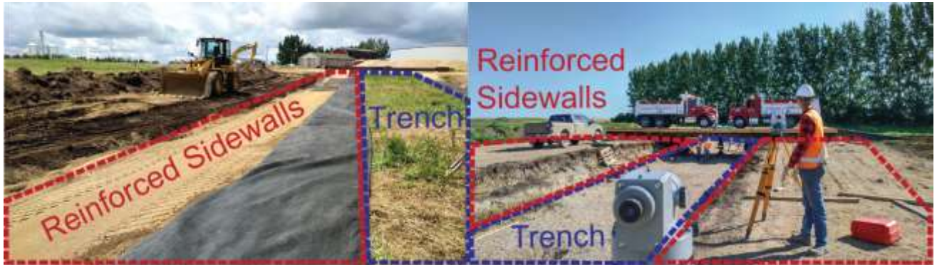
Figure 2: Construction of test pad trench and reinforced walls
