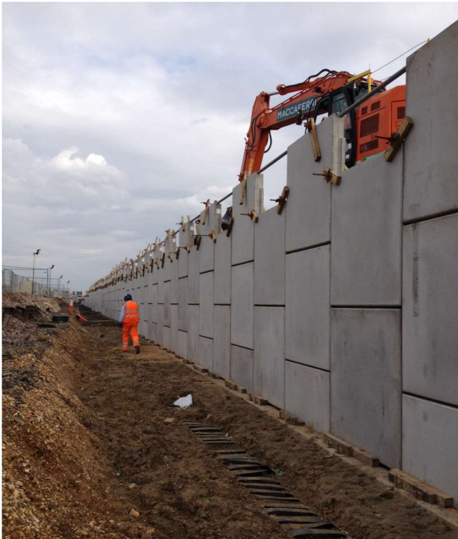
Figure 8. West ramp during the construction
