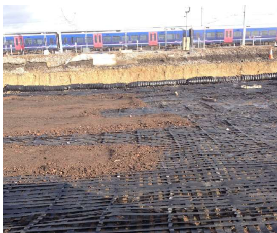
Figure 1. LTP geogrid placing
