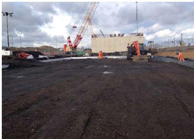
Figure 2. Soil placing on top of geogrids
