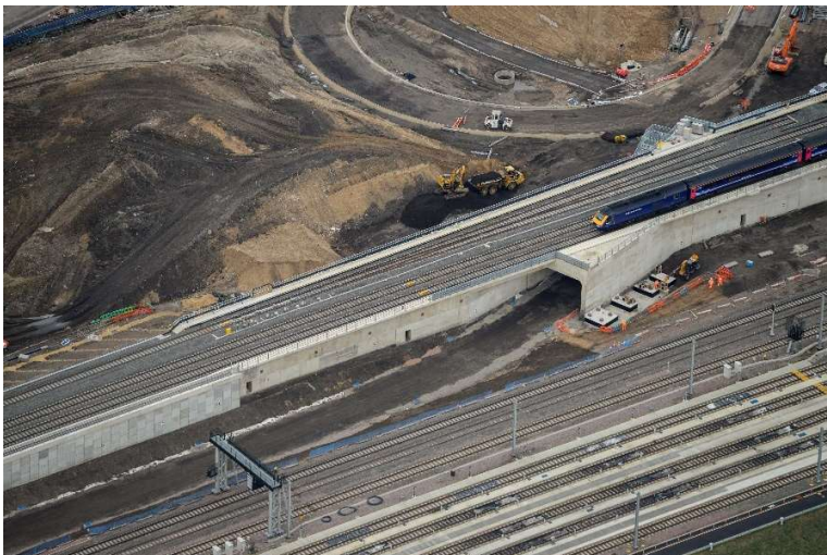
Figure 9. Aerial view of completed MSE structure
