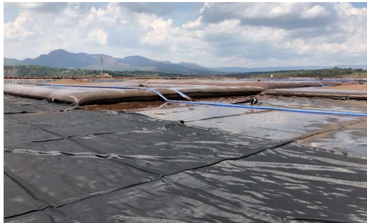
Figure 2: Woven Geotextile Tubes in operation during Phase 2 in Brumadinho, Brazil.
