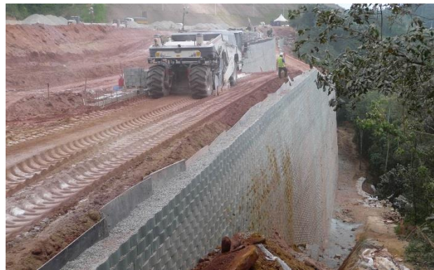
b) Execution of the earthwork near the top
