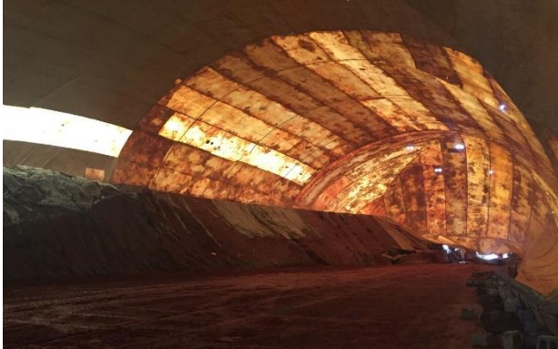
a) Execution of earthworks inside the roof (tent)
