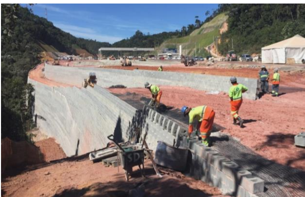
a) Final construction of the retaining wall
