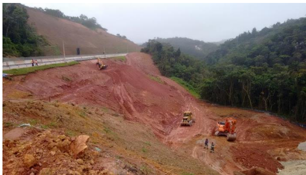
a) Temporary excavations in sub-section 1
