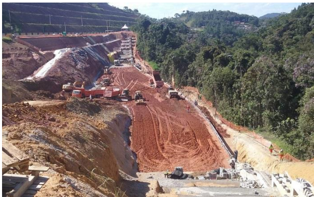
a) Execution of the earthwork near the base
