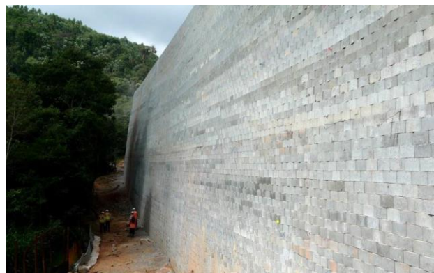
b) Face overview of the wall
