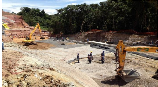
b) Execution of gravel and geogrid mattress
