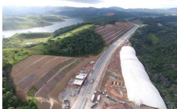
b) Overview of the site with cover (tent)
