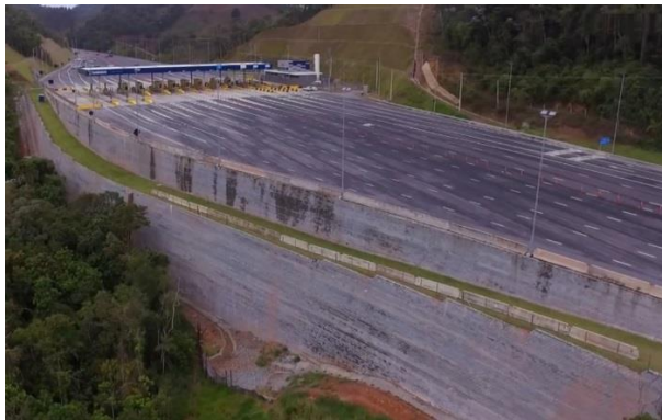
a) Final aspect of retaining wall and toll plaza
