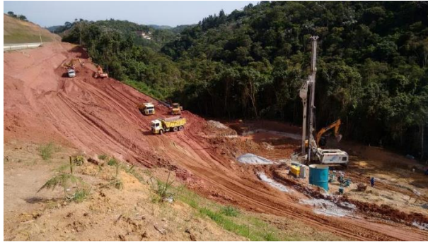
a) Execution of stone columns
