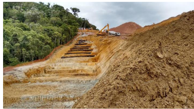
b) Temporary excavations and geogrids in sub-section 2
