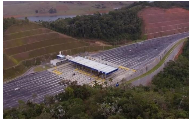
b) Toll plaza completed in operation
