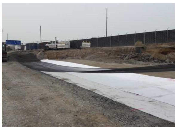
Figure 5. "Hanging" installation under pre-tension of the "bottom" knitted AR-geogrids
