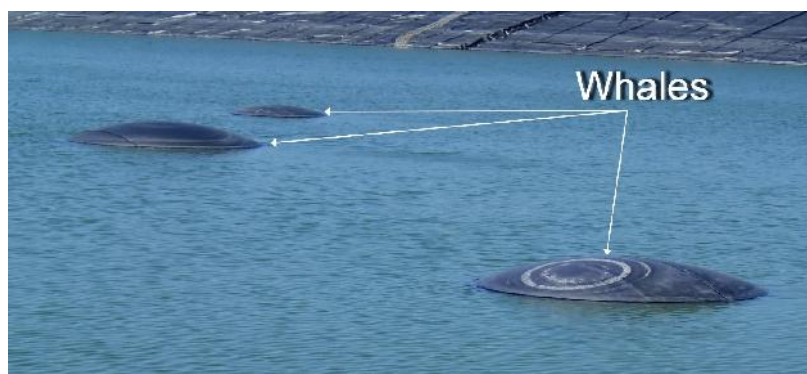
Figure 6. Examples of whales with trapped gas and liquid beneath the GMB
