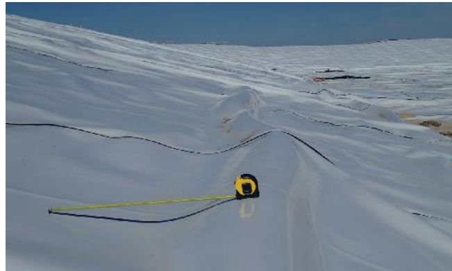
Figure 9. Wrinkle in white conductive GMB
