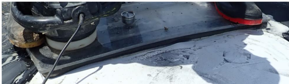
Figure 7. Photograph of vacuum box test
