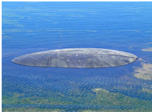
Figure 8. Photograph of typical geomembrane whale in pond
