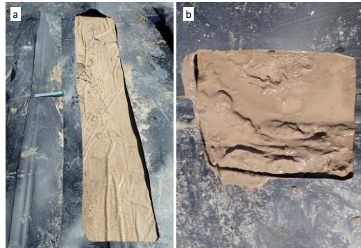
Figure 4. Inspection of subgrade at locations: a) Hole 1; and b) Hole 2.
