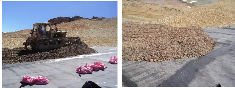
Figures 13. Pushing material of high grain size all along day whatever is the t°.
