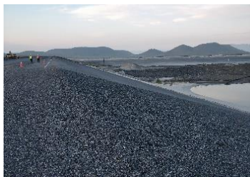
Figure 16. Peñasquito BGM lined - extension of the tailings dam
