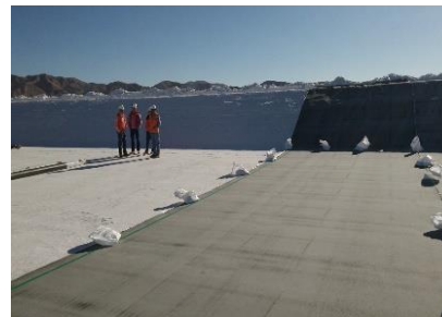
Figure 7b). No wrinkles of BGM despite being exposed at high temperature
