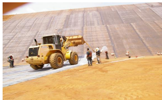
b) Site view of direct trafficability on BGM
