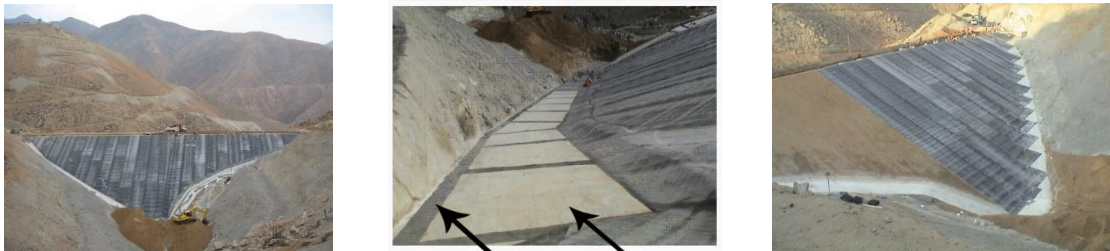
Figures 14. Cerro Lindo site, sealing BGM on concrete of abutments
