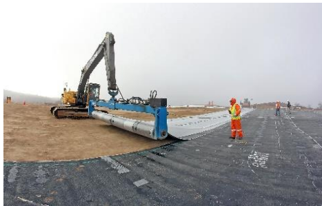
Figure 8. A 5.6 mm thick BGM deployed
