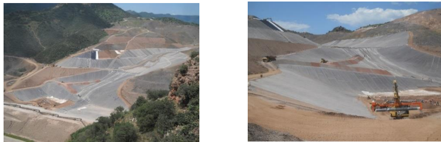
Figure 6. Dolores silver mine heap leach pad on a slope of more than 26°
