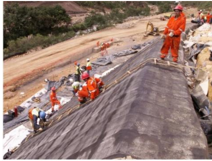
Figure 11. 1H:1V Slope installation
