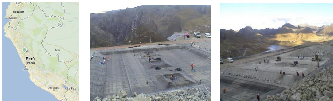
Figure 5. Antamina test waste rock pad at altitude 4,000 m
