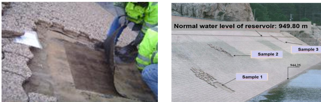
Figure 3. BGM Sampling Campaign on Ospédale dam (2007)
