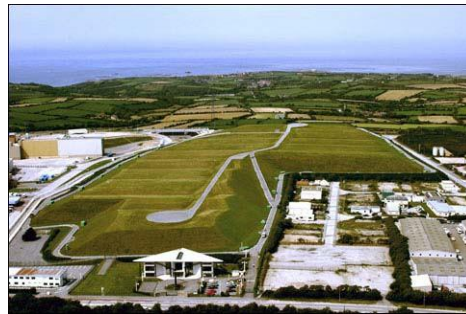
Figure 4. "La Manche" Radioactive Waste Storage Facility
