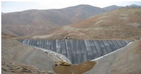
a) Work completed
