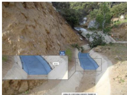
Figure 12. Contour canals, typical section
