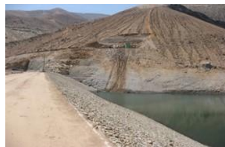
b) Dam in use after earthquake
