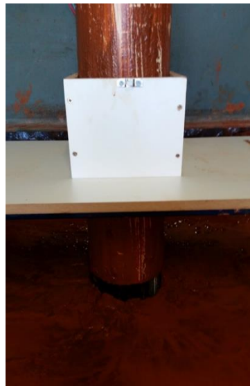
Figure 2. Use of the wooden casing for column driving.
