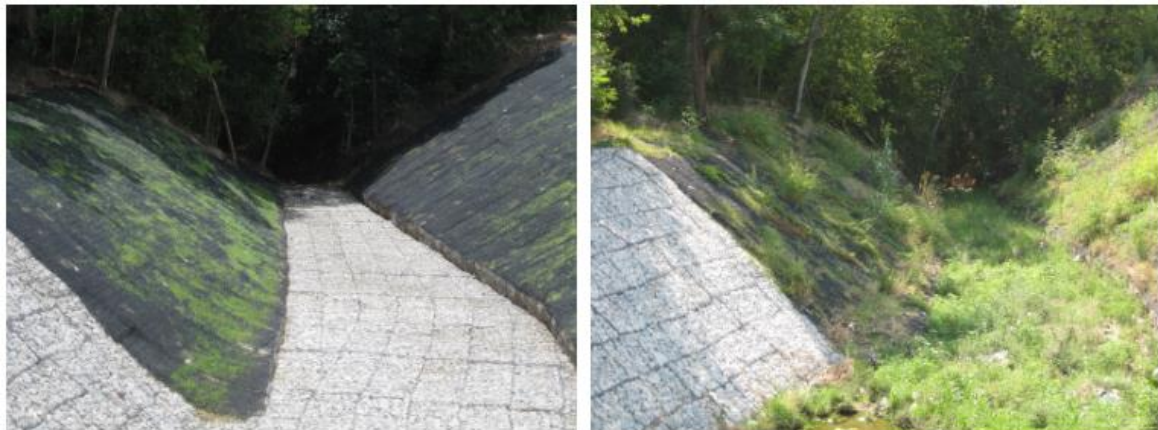
Figure 8. Vegetation growing on the DTWM reinforced geomat.
