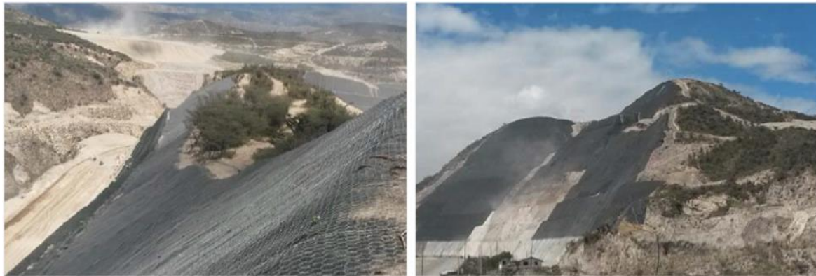
Figure 9. Installation of a geomat with DTWM reinforcement on a rocky slope.
