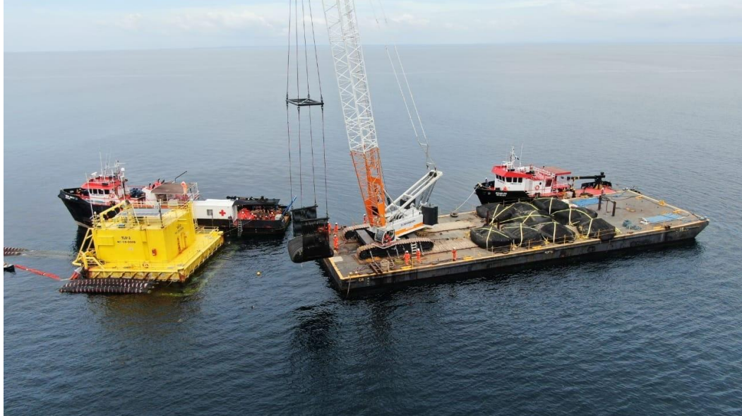
Figure 4 – Geobag Lifting Harness and Installation
