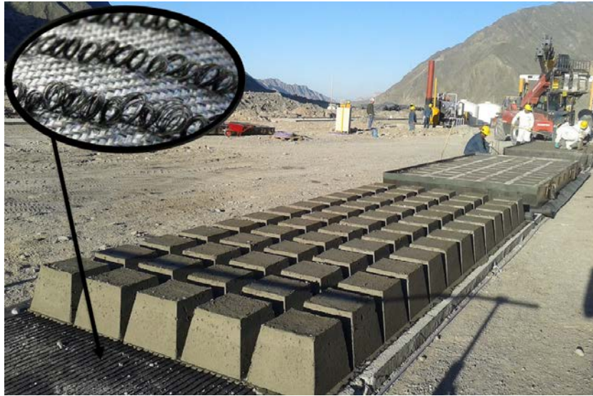
Figure 3. 30cm height concrete blocks linked to high-strength polypropylene loop matting fabric
