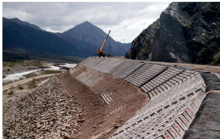
Figure 2. Concrete block mattress (CBM) in Punta Negra Dam
