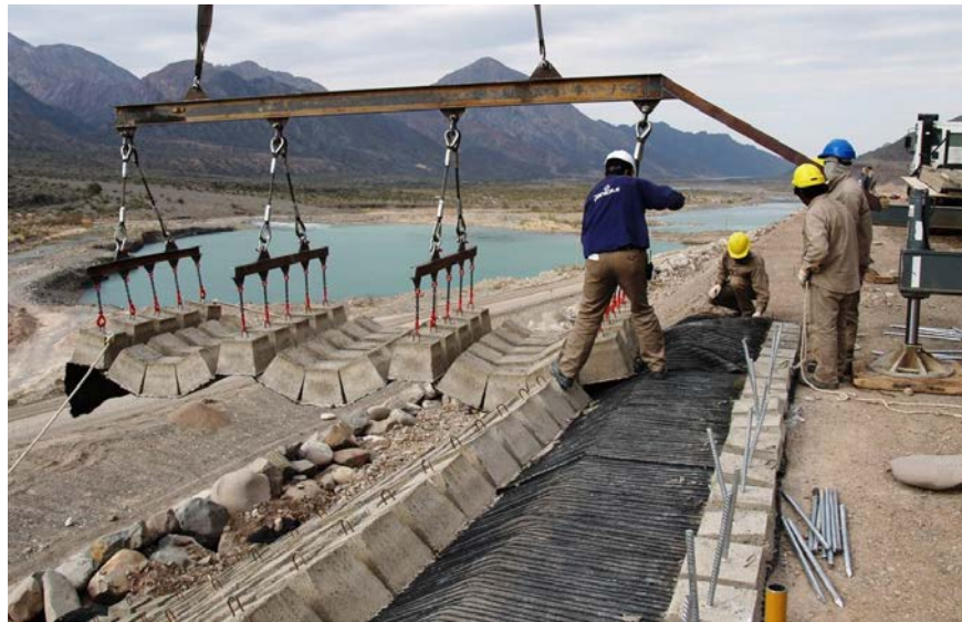
Figure 5. Steel pegs in every block
