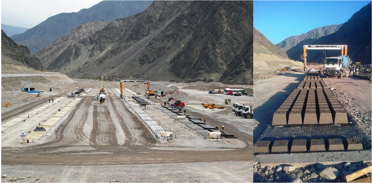
a) On- Site facility for precasted CBMs
