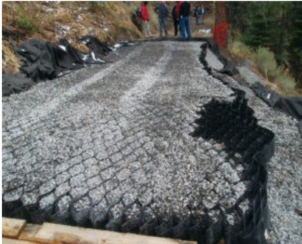
a) Geocell drainage structure
