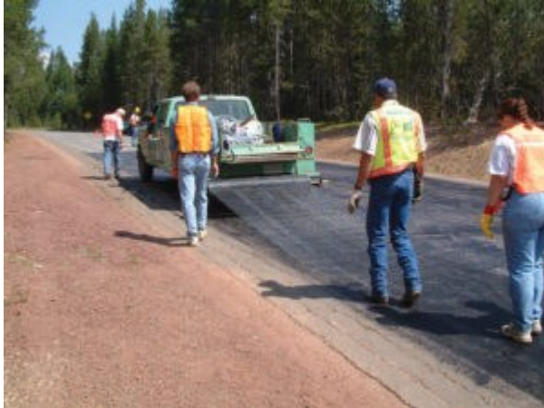
a) Reinforcement placement on a road
