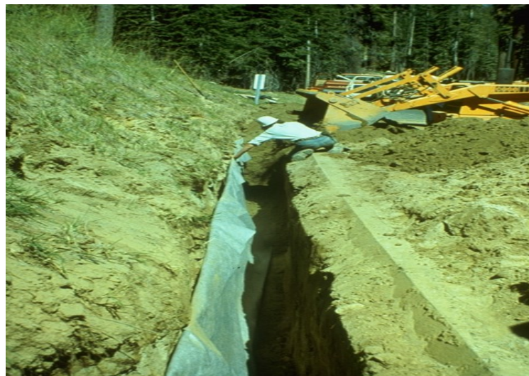
Figure 1. Installation of a geocomposite drain along a forest road in California, 1976.
