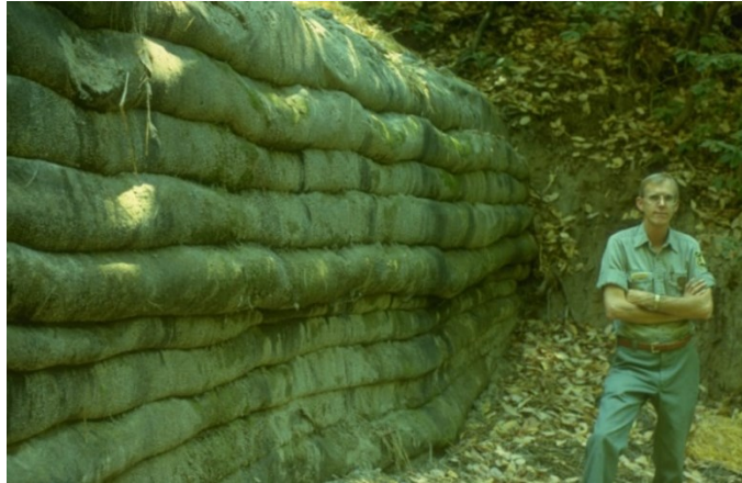
Figure 2. A geotextile wall constructed on a forest road in California in 1983.
