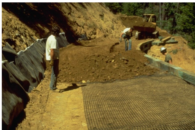
a) Timber-faced Wall
