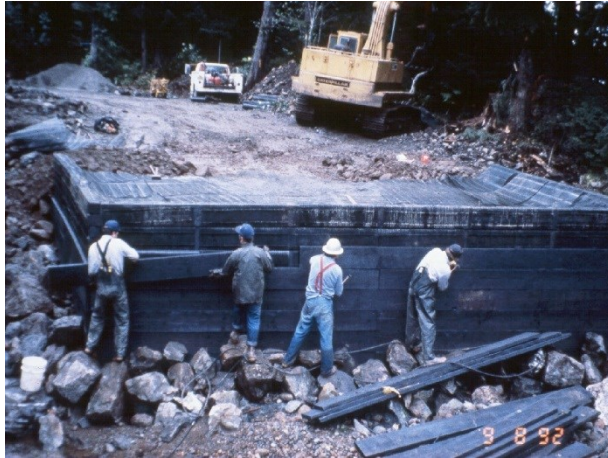
a) Timber-faced abutment
