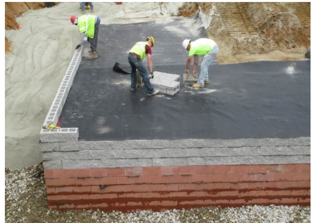
b) Concrete block-faced abutment
