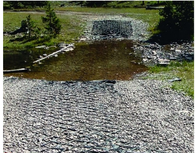
b) Geocell low-water crossing
