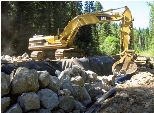
a) Geotextile filter behind riprap rock
