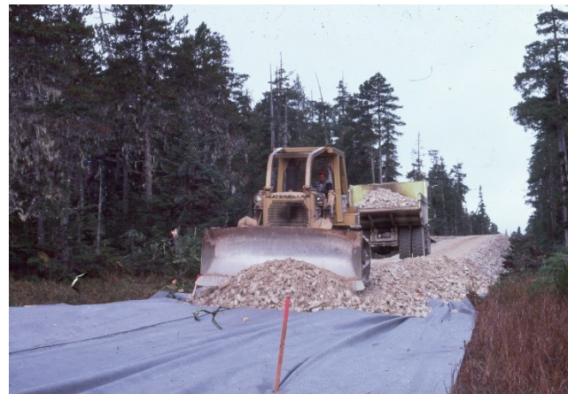
b) Geotextile over muskeg in Alaska
