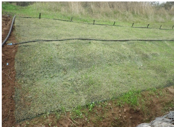
a) Erosion control netting
