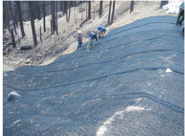
b) Geosynthetic turf-reinforcement mat on a slope
