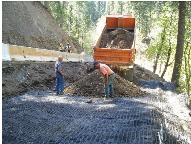
Figure 5. Construction of a deep patch road embankment repair project.
