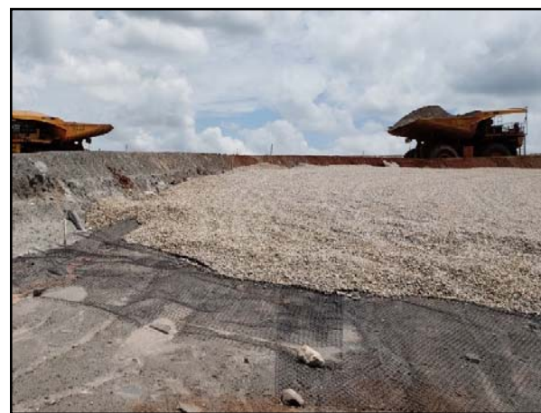
Figure 12. Installation of the final layer of gravel
