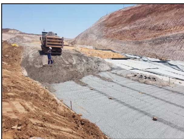
Figure 11. Installation of tailings on the rigid geogrid
