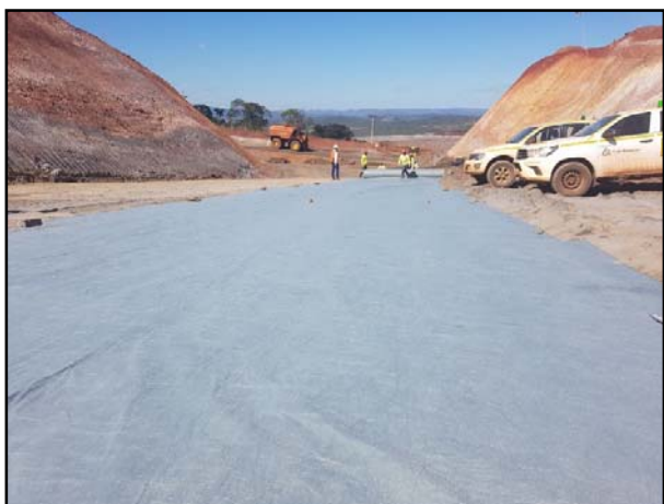
Figure 9. Installation of the non-woven geotextile of separation
