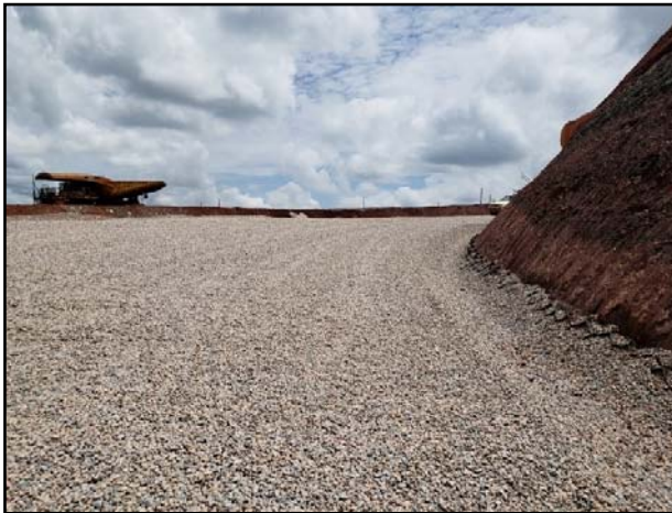
Figure 13. Reinforced mine road completed
