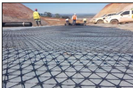
Figure 6. Multidirectional geogrid used in this project.
