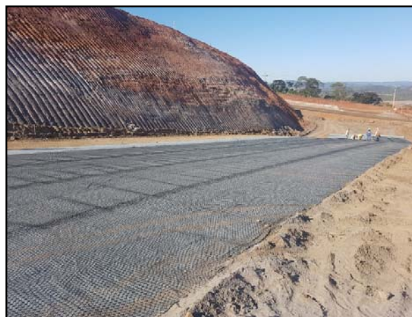
Figure 10. Installation of the first geogrid layer
