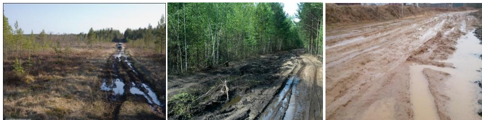
Figure 1. Temporary roads on soft soils.
